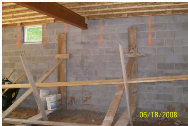
Bracing newly constructed masonry walls with substantial systems
