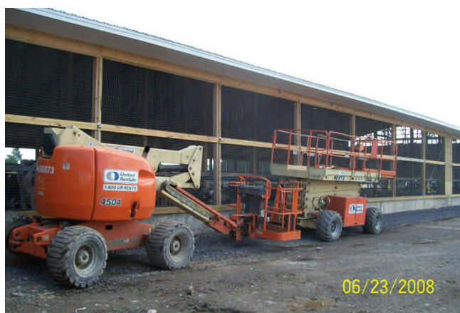
Rough terrain lifts on the job site.
