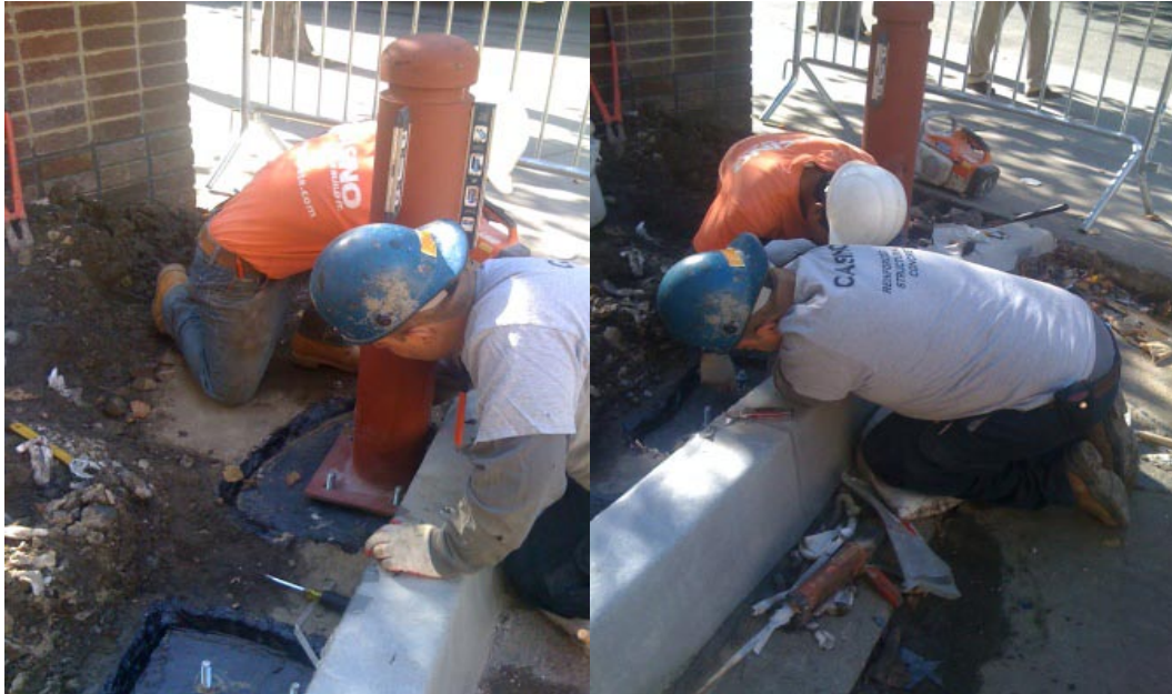
Before and After Temporary Sandbag Knee Protection
