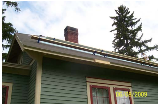
Roof Slides with Roof Jacks help to Prevent Falls
