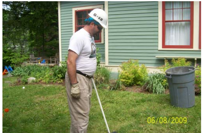
Maintaining an orderly jobsite is a "Best Practice"
