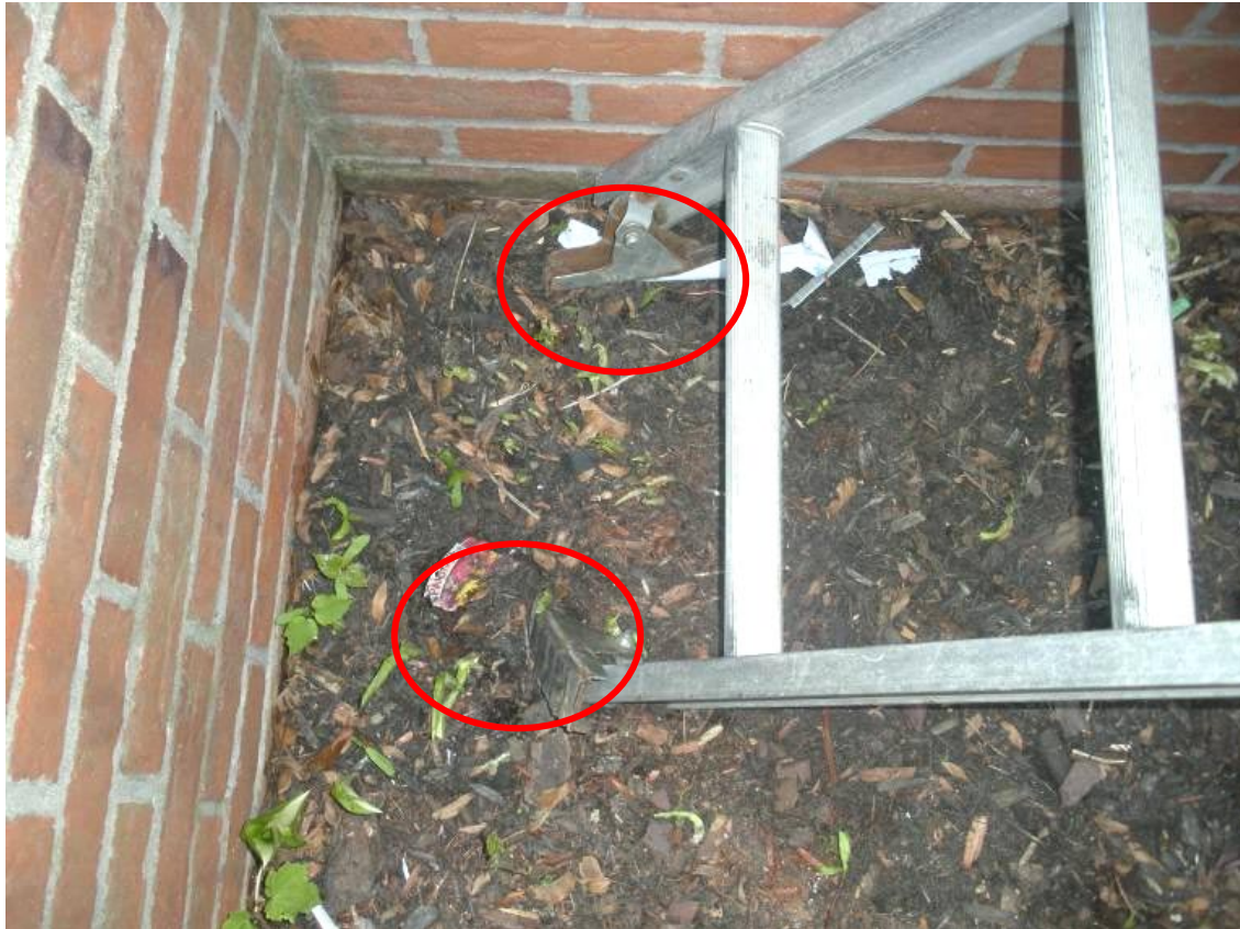
Ladder Shoes Bent and Unstable
