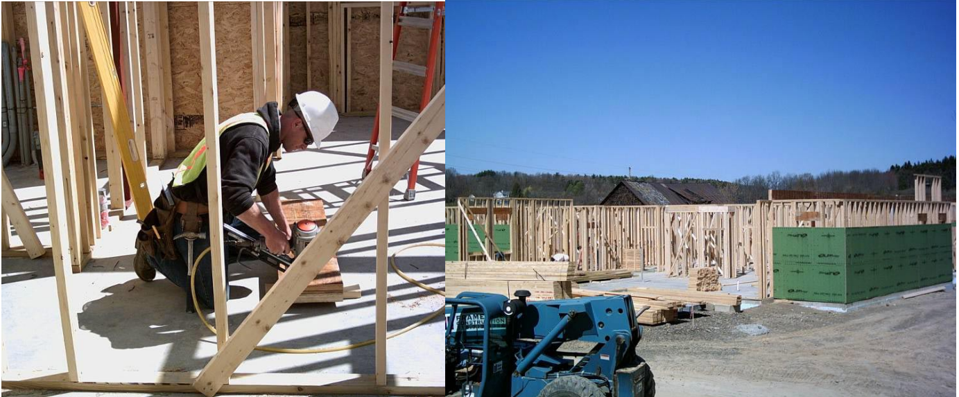
Framer Assembling a Door Header – Jobsite Picture
